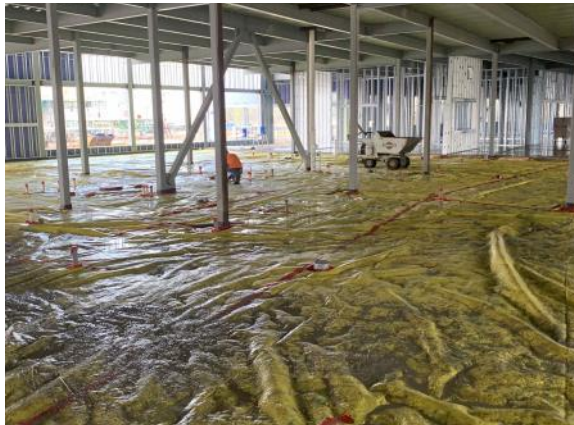
Concrete team preps for concrete floor pour in classroom wings (05/12/2022)
