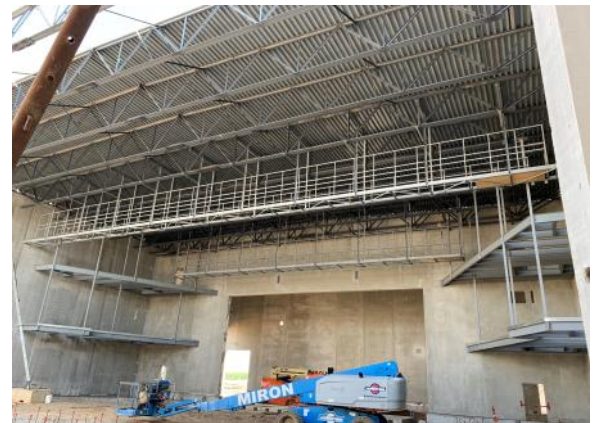
The steel catwalk structure over the auditorium is being erected (05/31/2022)
