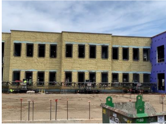
Exterior spray foam on the West classroom wings (05/06/2022)
