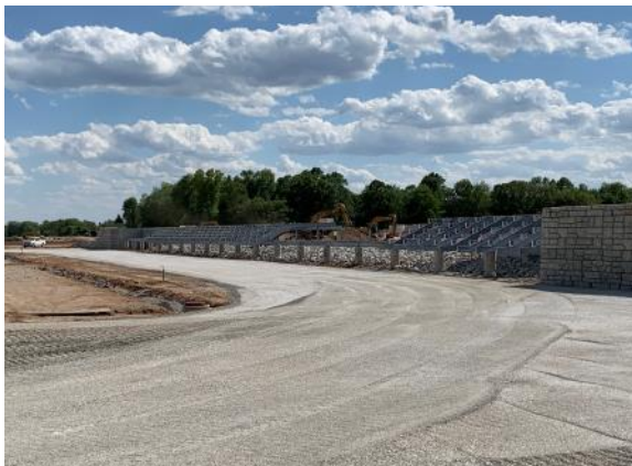
The grandstand bleachers start to be assembled (05/31/2022)
