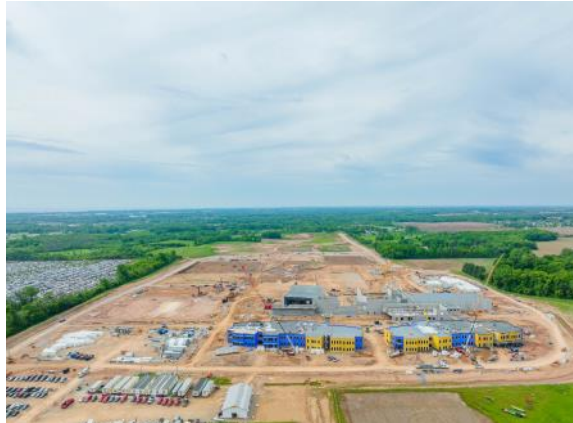
Looking South at the overall site (05/31/2022)
