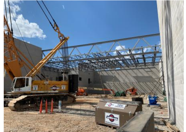
Large girder truss that spans the width of the competition gym and carries the weight of the roof (05/31/2022)
