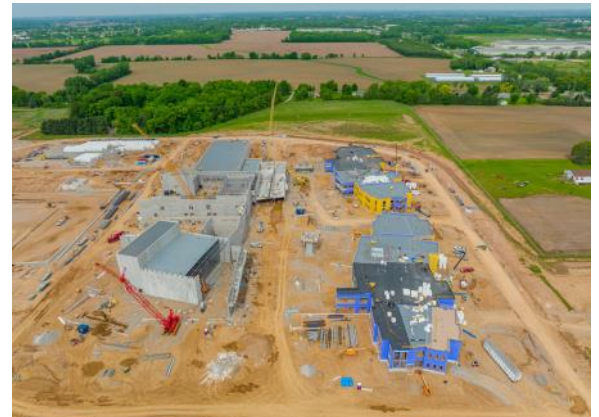
Looking West at the building (05/31/2022)
