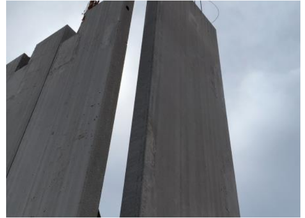
Precast panels in the auxiliary gym (05/06/2022)
